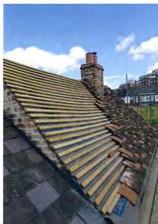
The clay tiled roof and chimney at number 22 in the course of repair
