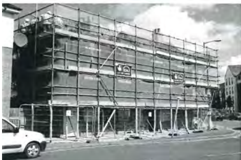
Visitors on top of the scaffolding at Weavers' Cottages
