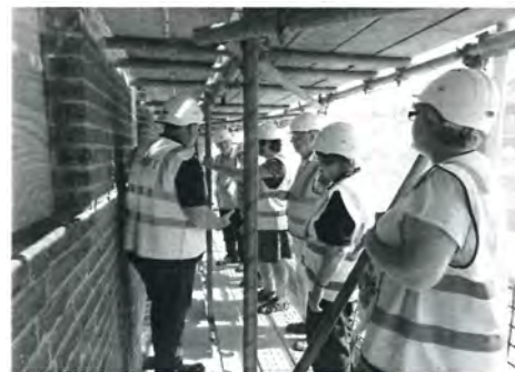
Visitors inspect the external brickwork from which the render has been removed
