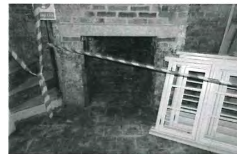
The original fireplace and quarry tiled floor at number 20
